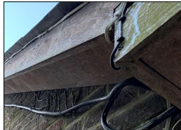
House verge and eaves (timber soffit and fascia boards) tight to wall surface.
