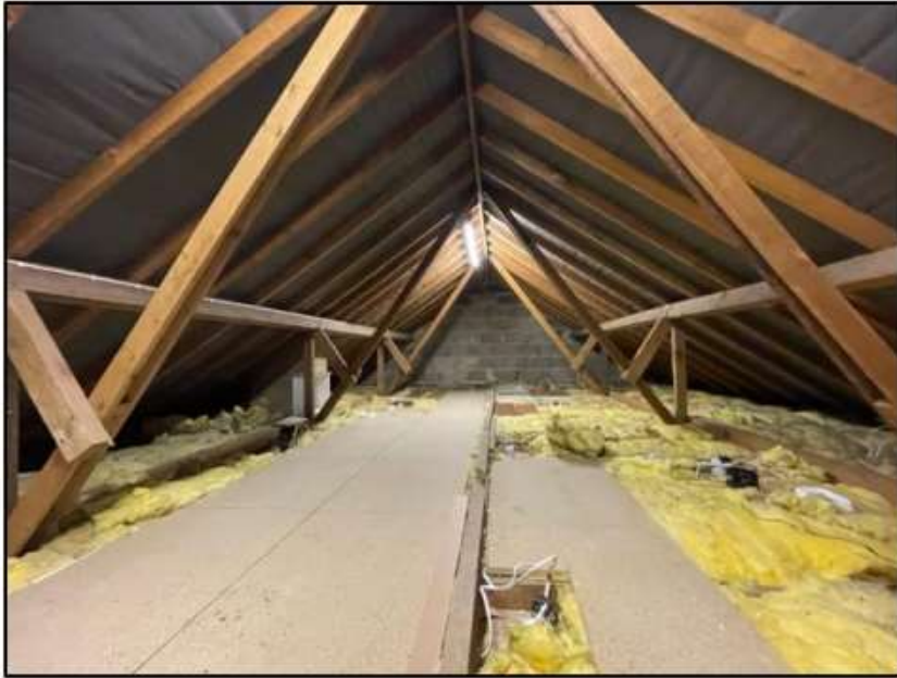
Loft space with close up of breather membrane
